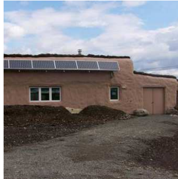
TNHA Projects From left: Five-plex and Northern Shelter in Anaktuvuk Pass
